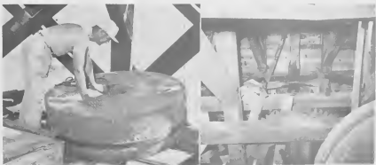
INSPECTING A grinding stone is J. Medendorp, one of four mill builders left in Holland, who came to Aruba un di e cuatro constructornan di molina cu a resta na te erect the mill. At right is a section of the wood Holanda, kende a bini Aruba pa para e molina. Banda gears which transmit power to grinding stones. drechi tin un seccion di e apartaton di palo.
